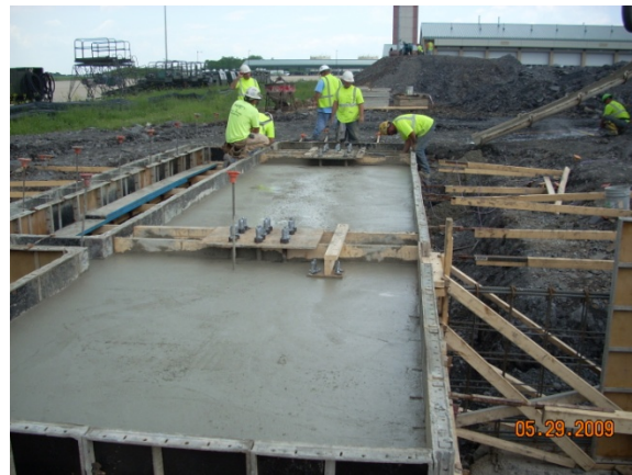
Pier Cap after placing
