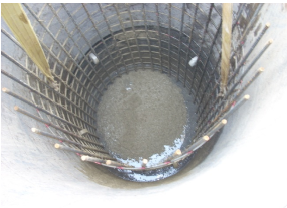
Caisson being poured
